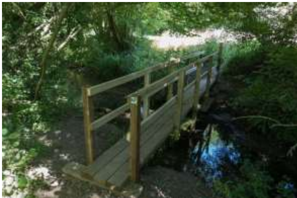
New bridge near Mill Lane
